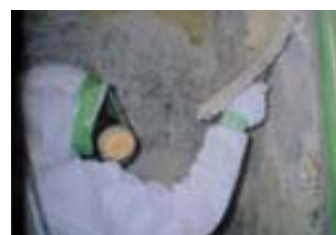
Asbestos removal
